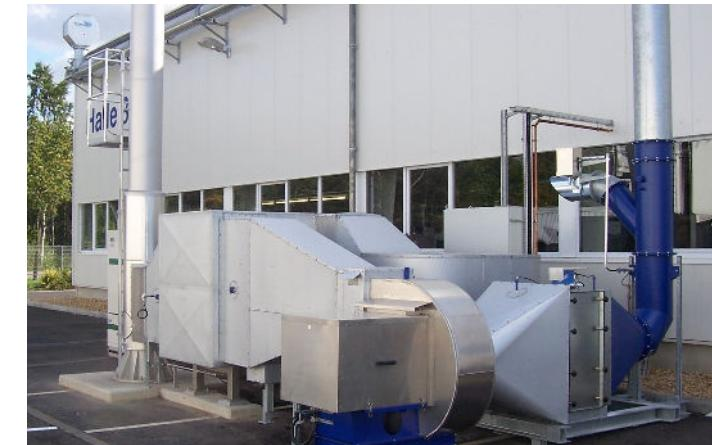
Catalytic incinerators are used to treat exhaust air, for example from the print, chemical and pharmaceutical industries as well as from various painting and coating systems.
