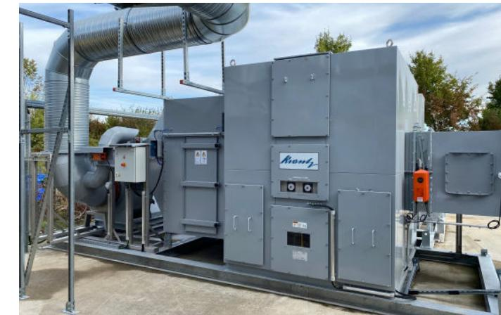
Due to the high VOC concentration in the desorbed air, the oxidiser is usually operated autothermally without additional fossil fuel consumption. Often, additional surplus heat can be used through the operation of an external heat exchanger.
