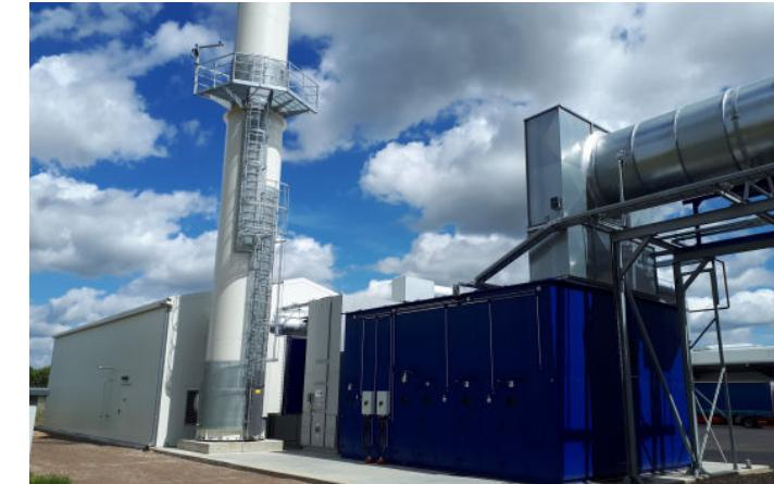
Even large exhaust air volume flows can be co-combusted in a microturbine if a concentration unit for exhaust air treatment is installed upstream as the first stage.
